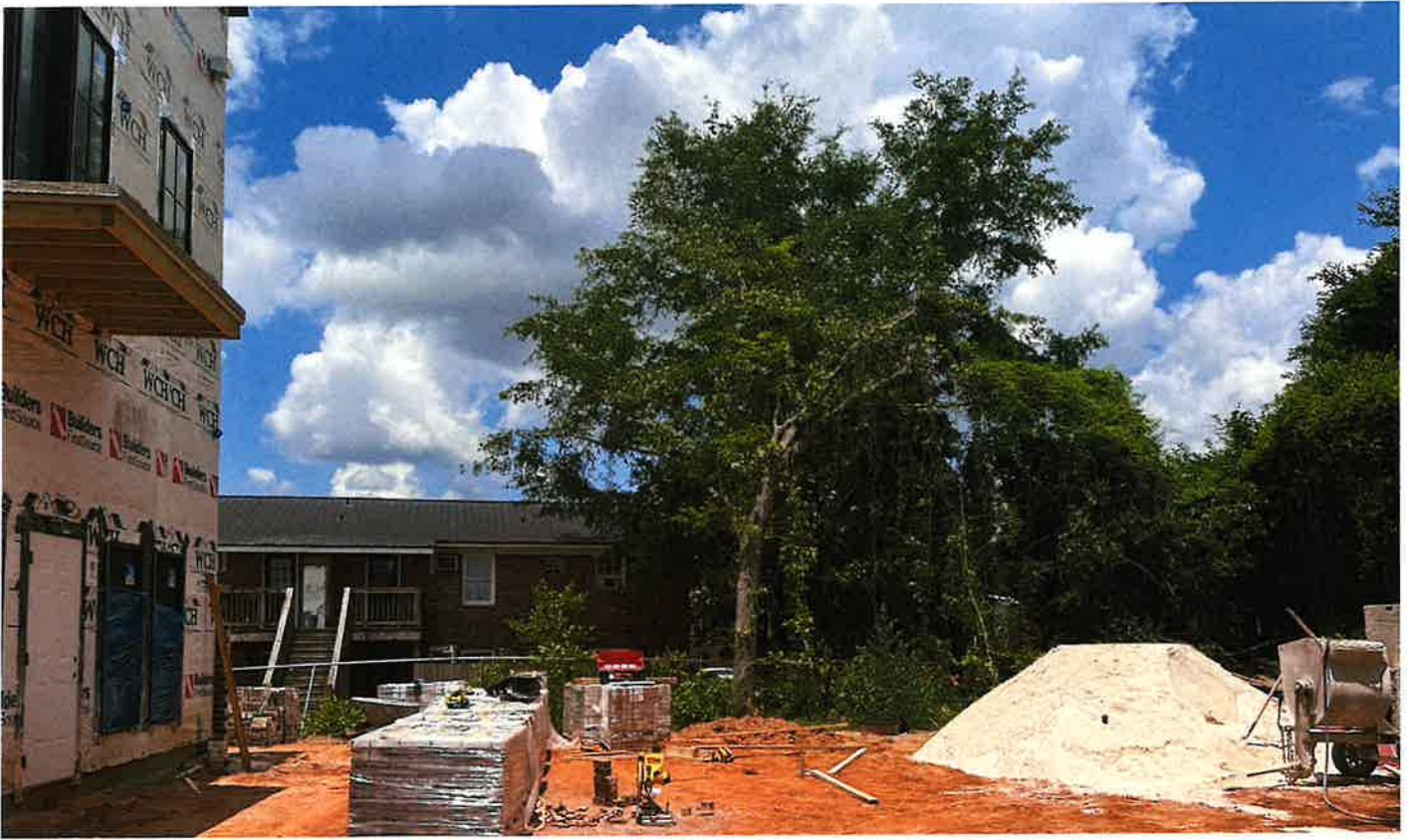
Views from subject property to adjacent property
